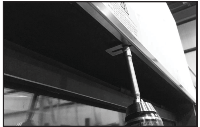
Figure 10.5. Install Trim Ring
