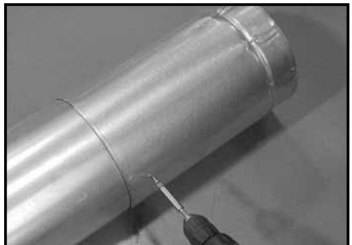
Figure 7.7 Screws into Slip Section
