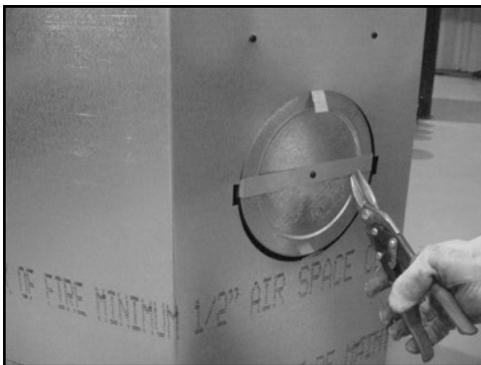
Figure 6.7 (Generic Fireplace Shown) Cut the metal retaining band and fold the sides out.
