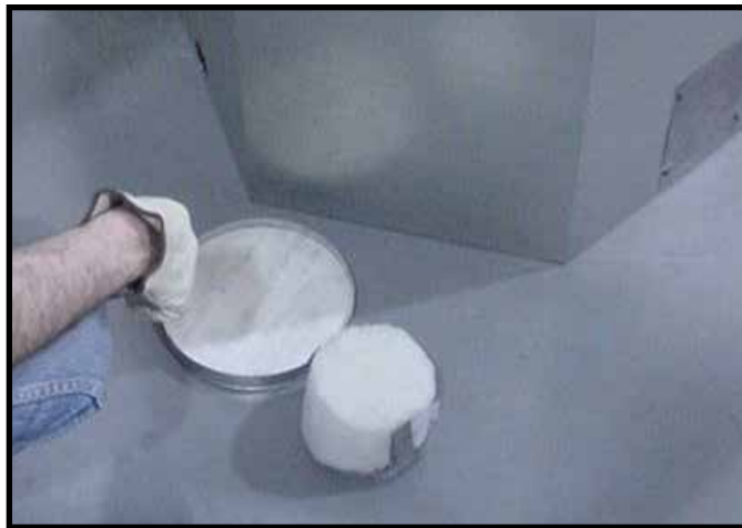
Figure 6.15 (Generic Fireplace Shown) Discard the seal cap, remove and discard the insulation basket. Note: Once the seal cap has been removed it CANNOT be reattached.
