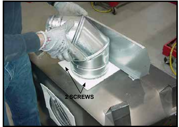
Figure 6.11 To attach the first section of vent pipe, make sure to use the fiberglass gasket to seal between the first vent component and the outer fireplace wrap. Use 2 self tapping screws to secure the gasket to the outer wrap.
