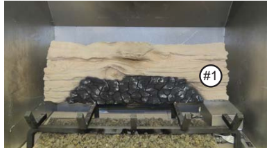
Place the rear log (#1) onto the 2 pins on the grate as shown.
