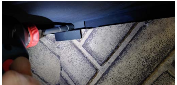
Figure 20.b Secure with the bracket using screw
