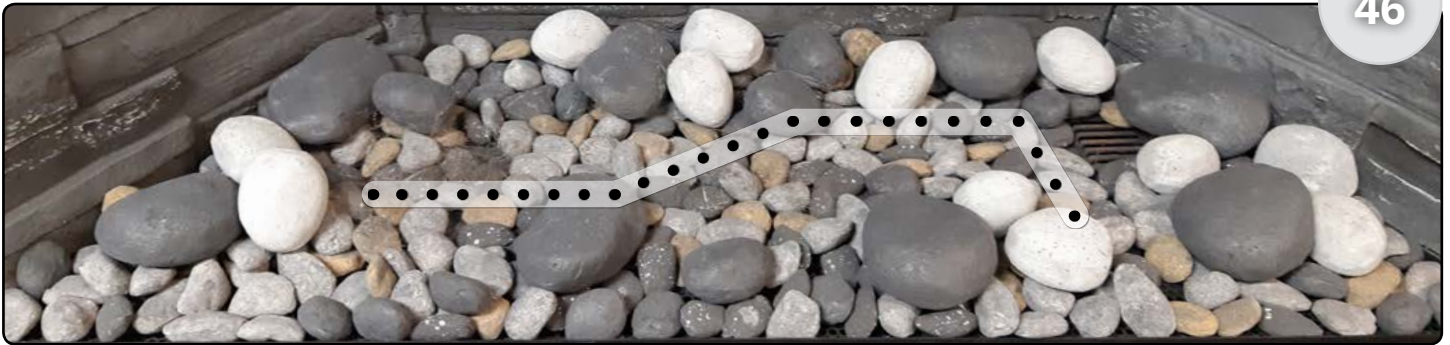
Figure 24.cc Completed Stone installation
