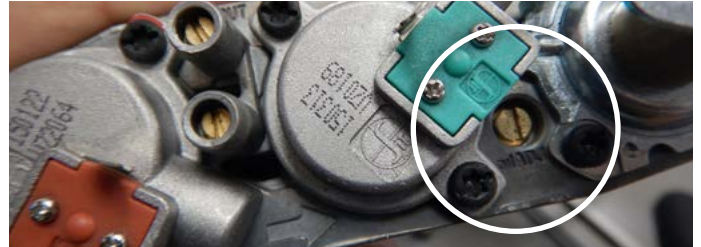
Figure 13.g Adjust pilot size
