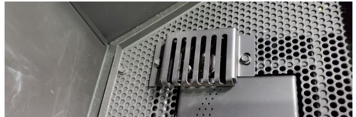
Figure 13. Removal of pilot cover
