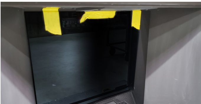
Figure 20.b hold it in place using masking tape
