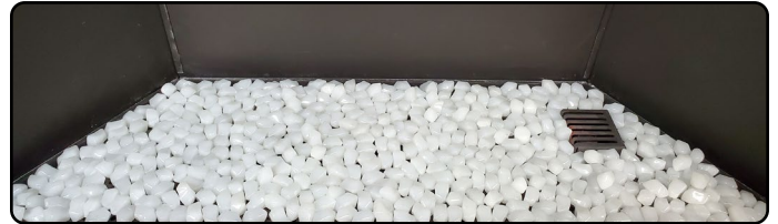
Figure 24.bb Completed firestone installation
