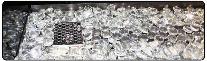
Figure 24.b Completed firestone installation
