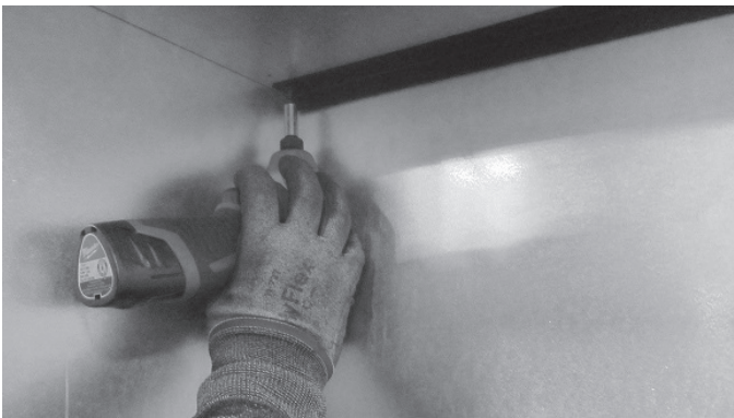
Figure 7.2 - Remove Rear Black Magic Glass Bracket
