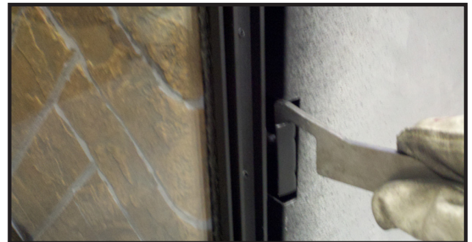
Figure 11.7. Securing Side Glass Clips
