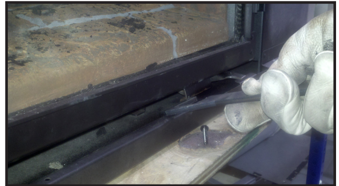
Figure 11.2. Glass Clip Tool Location
