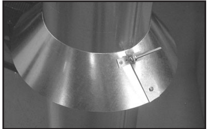
Figure 7.12 Insert Bolt into Brackets
