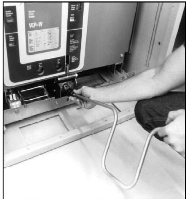
Figure 4-6 Engaging Levering-In Crank
