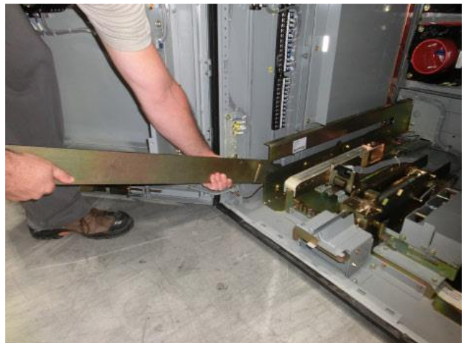
Figure 4-2A Insertion of the Drawout Extension Rails
