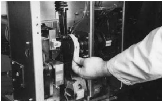
Figure 6-16 Remove Marked Masking Tape From Cam
