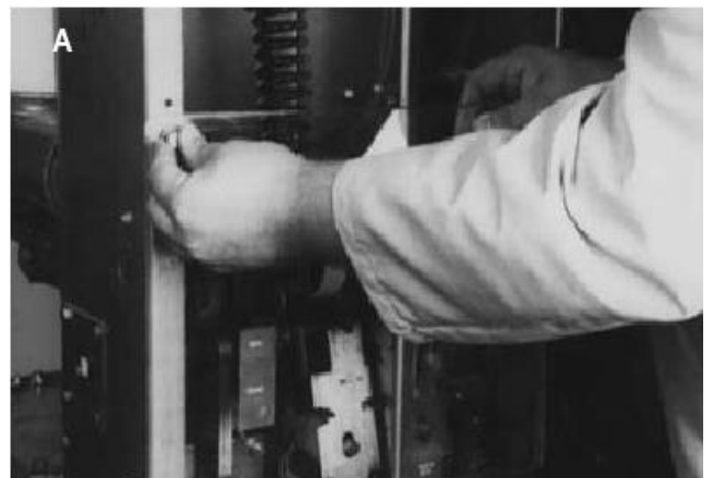
Figure 6-9 Attaching CloSure™ Test Tool at Hole “A”
