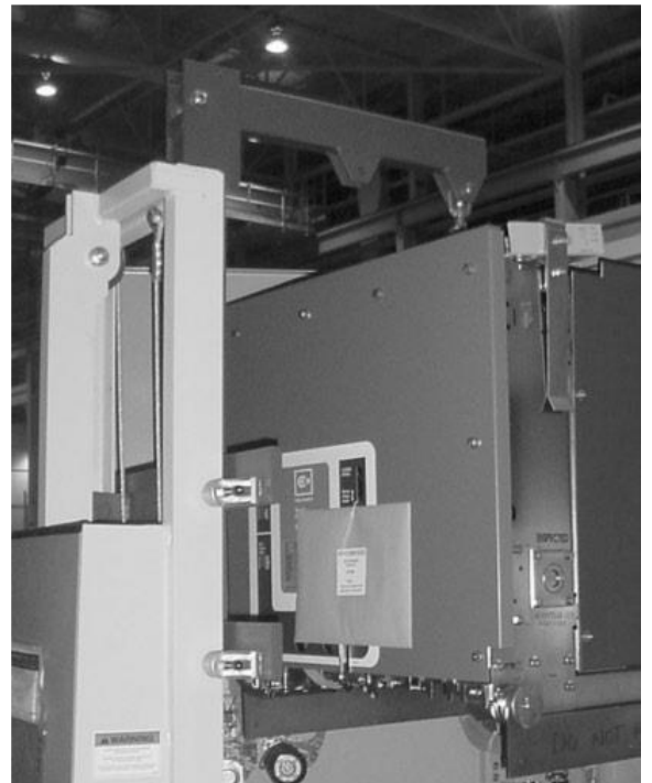
Figure 4-2B Lifting and Setting the Breaker in the Housing
