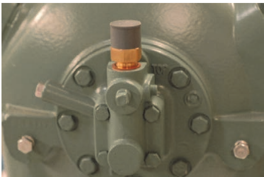
Fig. 23 — OPSS Sensor Installed
