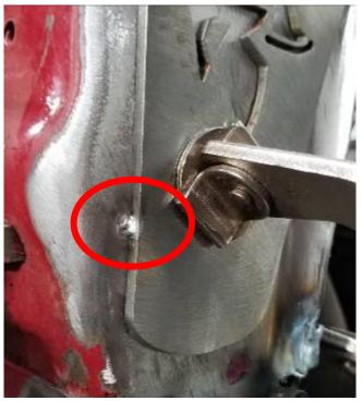
• Next, tack weld the tower bars to the frame bars
