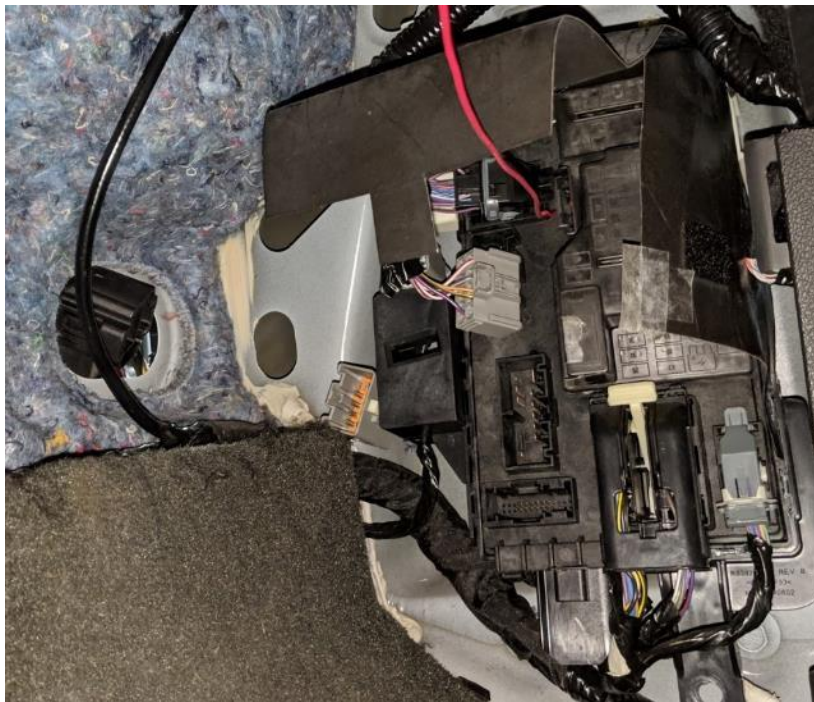
(View of junction box from passenger floorboard)
