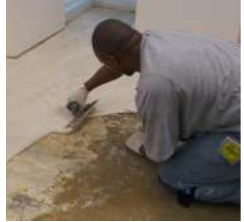
Apply adhesive to floor following manufacturer's recommendations
