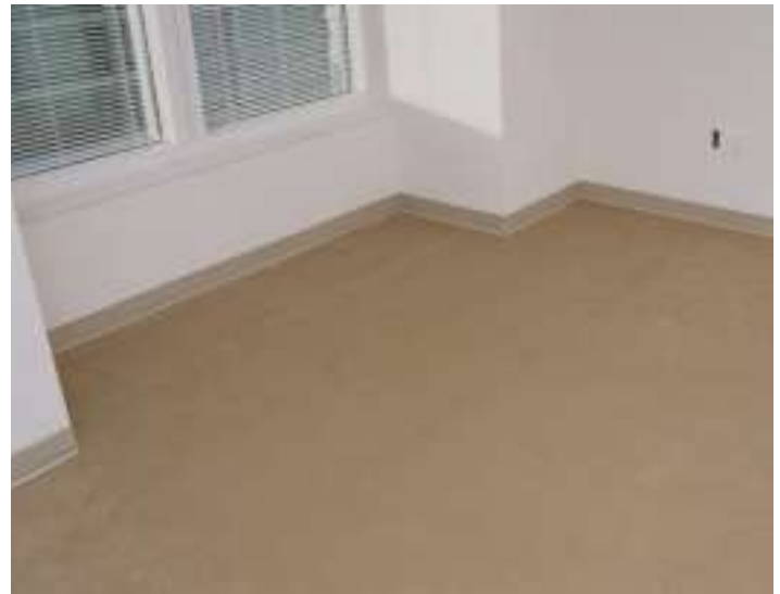
Prevent traffic over carpeted area for a minimum of 24 to 48 hours after installation
