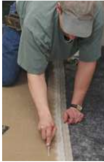
Dry-fit carpet according to layout plan
