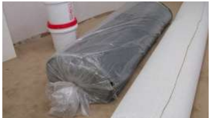
Acclimate materials for 48 hours prior to installation
