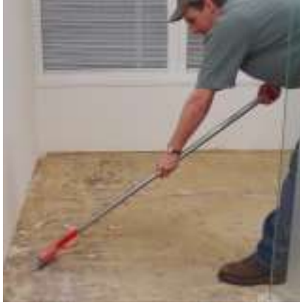
Start with a clean, dry, and smooth floor
