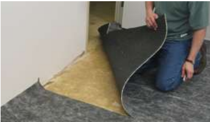
Cushion seams should have no compression or gaps
