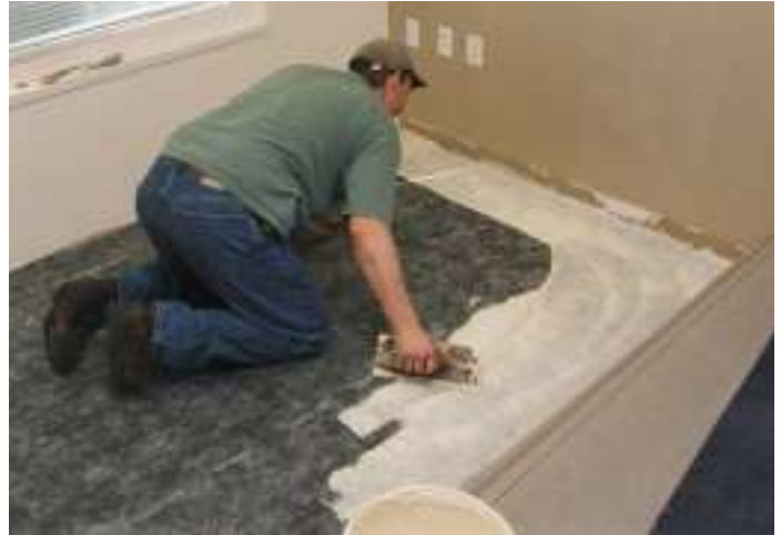
Apply adhesive to cushion following manufacturer's recommendations
