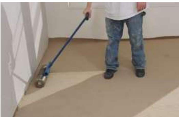
Roll in both directions to promote complete adhesion
