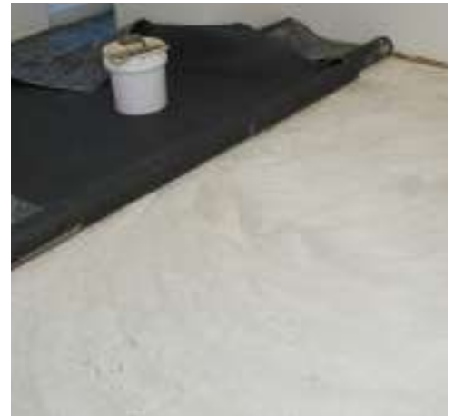
Proper open time is critical for a successful installation
