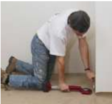
Install carpet and trim in
