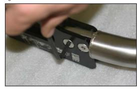
\*Do not force bolts, if you need to, loosen pre-installed bolts to align threaded backing plate correctly. Loosely install all bolts before final tightening.
