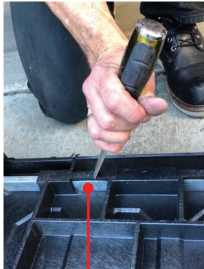
Chisel plastic from pilot holes if needed.
