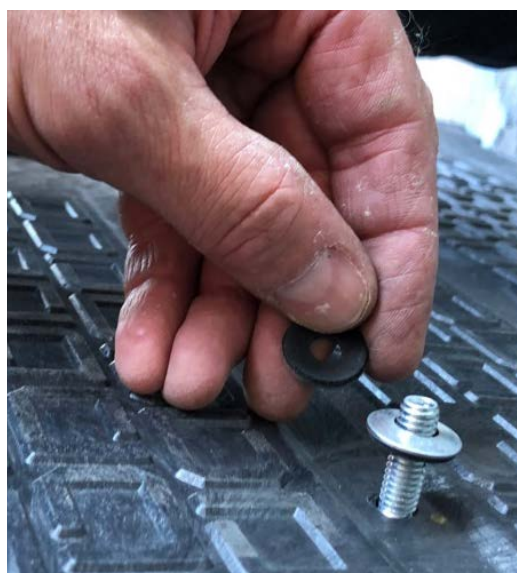
RUBBER WASHER [RUBBER SIDE AGAINST DECK PANEL]
