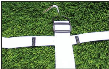
Step 6: Apply crossing lines as desired. The perimeters are labeled every 2.5 yds. Use these marks as guides for your lines, anchoring them across the perimeter lines on the outside of the playing area.
