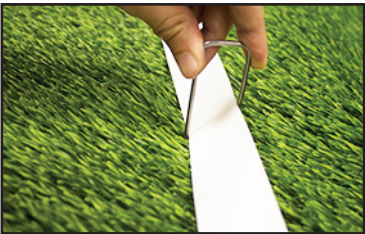
Step 5: To finish, place a wicket at the mid point of any line.
