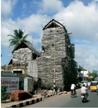
Andamiaje Construction scaffolding Pondicherry, Tamil Nadu, India
