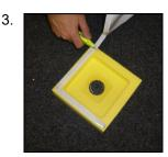
Use the butyl tape provided to make an airtight seal around the base of the unit. lf necessary, two layers of tape can be applied if the floor is uneven (see below for information about replacement supplies).
