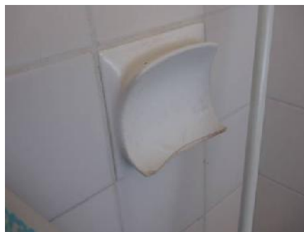
This broken soap dish in the shower could cause injury and needs to be replaced.
