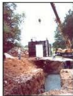
Shelter being lowered into wet cement.
