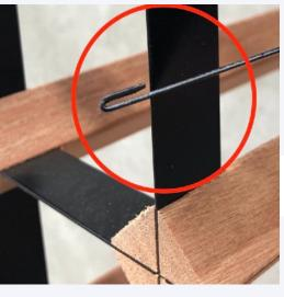
Hook the wall bracket to the front frame of the wine racks
