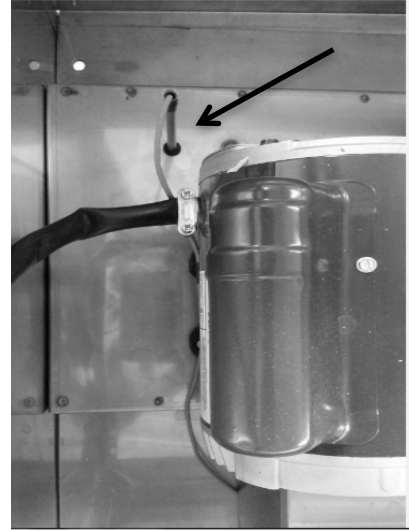
Figure 2 Crusher Probe Location
