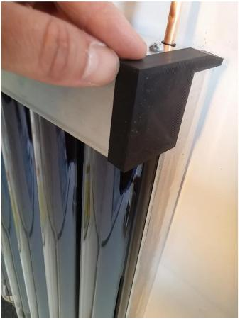
8) Push the plastic end caps onto the open ends of the frame top.
