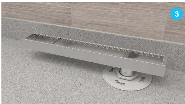
Step 3. Insert the drain channel into the threaded nipple.
