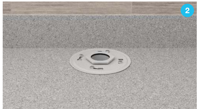
Step 2. Mark the center of your shower and screw threaded nipple into the drain flange, adjust to desired height.
