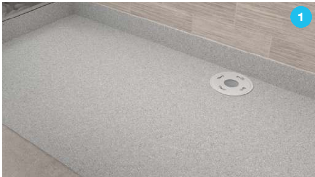
Step 1. Have your shower area ready, waterproofing installed and tested.
