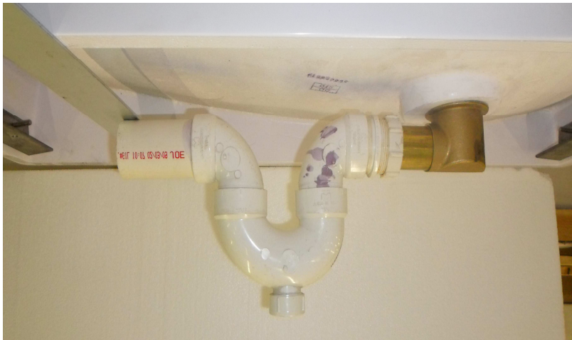
Tub shoe and P-trap connections. Suggested pipe is 1-1/2" diam
