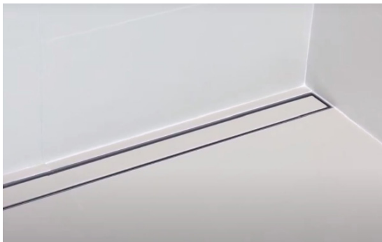
Off the Wall Installation
