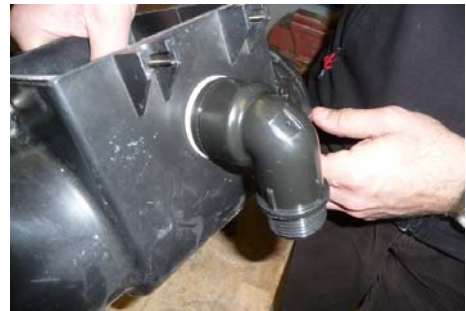
Fig. 4: Installed 90° connection bend
