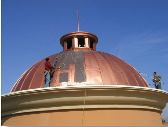
Left: Cabazon Outlet Mall - Cabazon, CA. Coated with Copper B Metal Coating.
