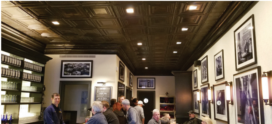
Below: Metal Coatings and patinas on ceiling tiles by Heartland Construction, Chicago, IL
