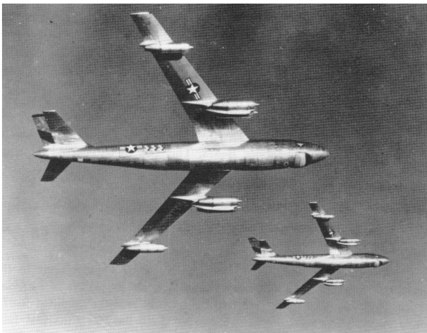
Two B-47Bs, equipped with 6 J47-GE-23 engines.
