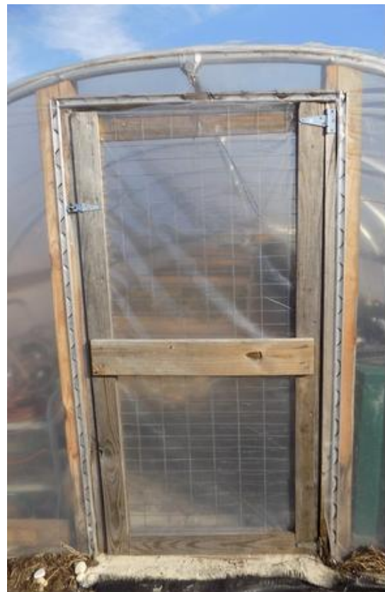
This door uses chicken wire and plastic for the door. Our instructions call for polycarbonate roof panel. Use whichever you prefer!
