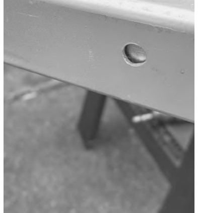
Door Frame Corner Showing outside 1/4" opening
