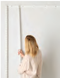
Screw the Top track into the wall, leave minimum 15 mm gap to the ceiling or cornice. For the best visual impression, we recommend to mount the Top track at the height where you want to place the top shelves. Hang the hang standards on the Top track.
