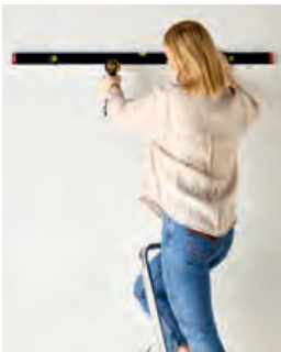
Screw the Top track into the wall, leave minimum 15 mm gap to the ceiling or cornice. For the best visual impression, we recommend to mount the Top track at the height where you want to place the top shelves. Hang the hang standards on the Top track.
