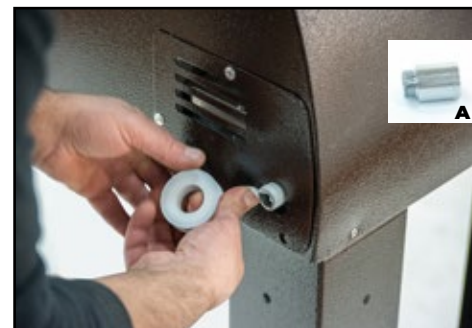
1. Insulate the oven gas connection with Teflon tape (A) and screw in the gas hose.
