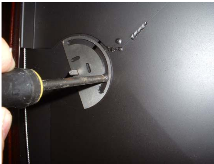
Photo 14: Restrictor Fully Opened (no restriction)
