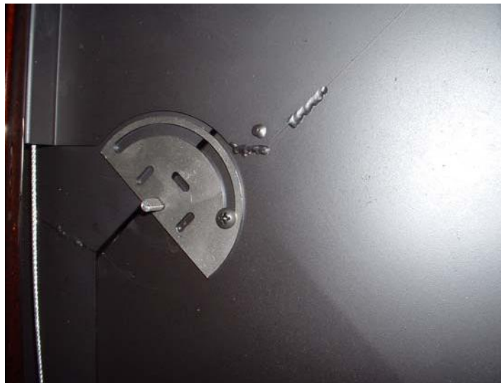
Photo 13: Restrictor Fully Closed
