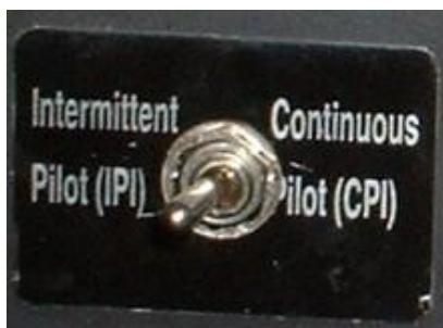
Photo 2 – Pilot Mode Switch
