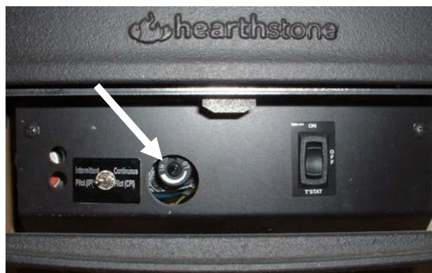
Photo 39 – ST Valve Output Control
