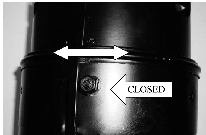
Figure 6: Restrictor in closed position
