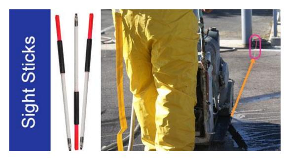
Sight sticks can be used by experienced saw cutters. Simply mark the four corners of the loop with the metal sight sticks which are used as targets to guide the saw-cutting machine. Go straight from laying out the loop to cutting with these tools.
