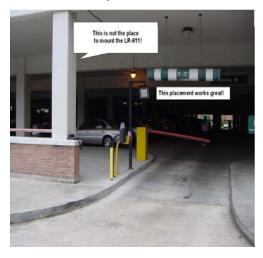
In this instance, the fact that vehicles were turning through the read zone meant poor performance when the reader was mounted on the white post. Once the reader was moved back closer to the operator, it worked much better!
