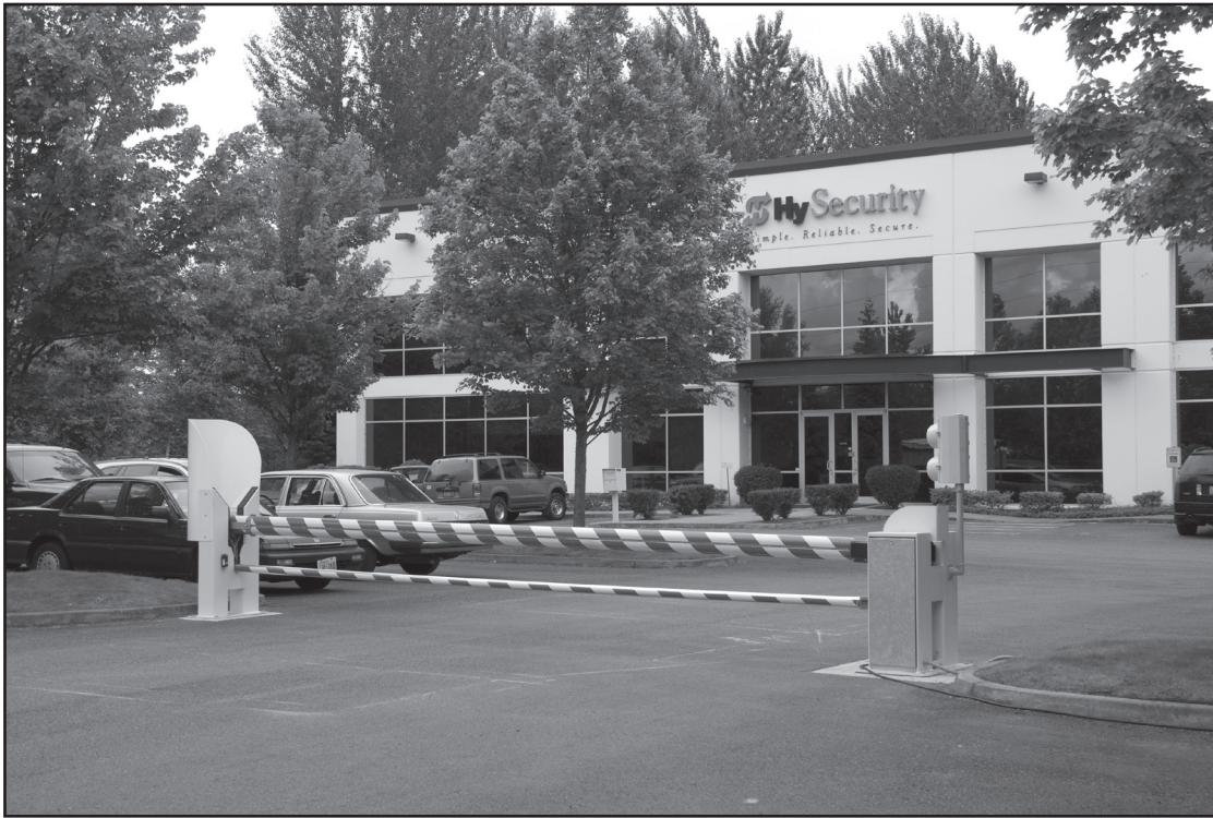
HySecurity Gate, Inc. Headquarters in Kent, WA
