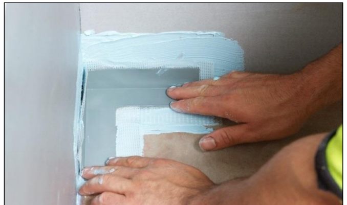
Installing Elastoproof Prefabricated Corners
