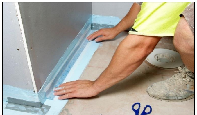
Installing Elastoproof B50 Bond Breaker Joint Band
