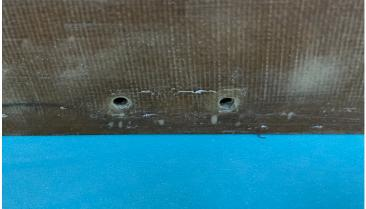
Holes drilled through mold to attach the overflow. (use hole template provided)
