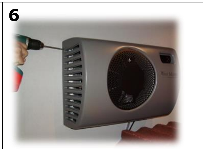
Refit the cover on the Winemaster and tighten the 4 screws
