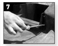
Attach liner bracket and liner to waterfall weir by installing 4 tack screws **halfway** into each corner. (Front of bracket has recessed screw holes.)
