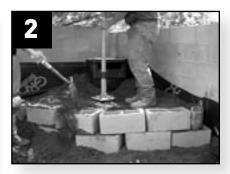
Use soil excavated from the pond to create a runway for the waterfall. A retaining wall of blocks can be used to provide shape and underlying structure.
