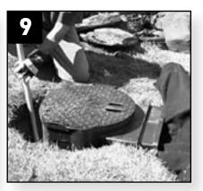
Backfill around the Skimmerfilter™ with the lid in place. Use moist sand or pea gravel or, if unavailable, gravel and loose soil (free from clumps). Hand pack every two or three inches. Do not over compact. Lightly moisten the backfill to aid in settling.
