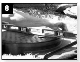
Level the unit front to back and side to side. Make the front edge %" lower than the back edge. Check water level once again.
