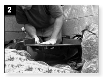
Slide waterfall weir into place. Ensure that the weir seal is firmly compressed between the weir and filter chamber, with flat side of seal facing toward the filter body.
