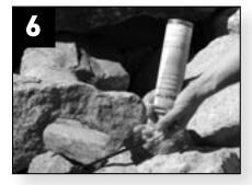
Use Savio Black Foam<sup>™</sup> to fill gaps in the rocks, preventing water from disappearing beneath and between them.
