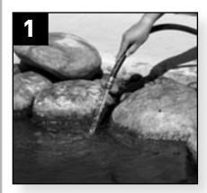
Fill the pond using a garden hose. This will allow you to accurately determine water level on all sides before proceeding with installation of the Skimmerfilter.™ Water level should hit partway up the coping stones. Verify that the water level is a few inches below the edge of the liner on all sides.
