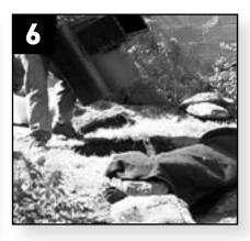
Place the Skimmerfilter™ in the hole. Check to make sure the intended water level meets the skimmer 3¼" inches below the top of the neck. Adjust up or down by adding or removing dirt.
