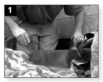
Pull liner over the face of the Livingponds Filter.™ Cut liner to shape of opening, as shown.
