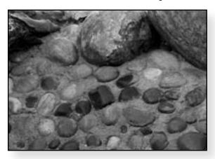
To create a safe, durable, easy-to-clean decorative rock bottom pond, press river stone halfway down into a fresh 2" layer of cement on the shelves. Build up and stabilize vertical stone walls with mortar.
