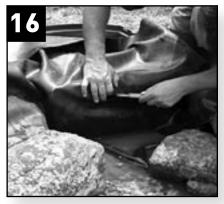
**A)** Make a 3" wide incision through the centered liner ¾" below the top of the Skimmerfilter™ opening.
