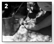
Connect hose to back of Waterfall Weir™ and tighten with hose clamp.
