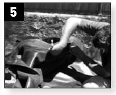
Mark position of the weir opening by rubbing the liner with a hard object such as a screwdriver or a blunt scissor edge.
