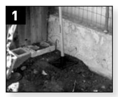
Level the soil in the area where the assembly is to be placed. Use blocks to add height to the waterfall.
