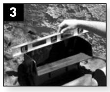
Place the Waterfall Weir™ and level the unit front to back and side to side.
