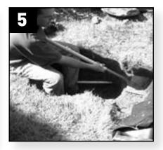
Dig a channel 7" below the water line, measuring 24" wide, from the hole to the pond. The Skimmerfilter™ neck rests on this channel. Compact and level the bottom of excavation. Do not dig too deeply or the soil may settle unevenly.
