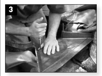
Insert and gently tighten the four large sheet metal screws into the holes in the waterfall weir. Do not over tighten.
