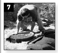
Verify that the face of the Skimmerfilter<sup>™</sup> is flush with the back wall of the lined coping shelf. Adjust placement, if necessary.
