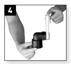
Put teflon tape onto 90° elbow.
