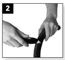
Cut to length leaving 12" of excess Kink Free Hose™ inside the Skimmerfilter.™
