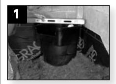
Level the soil in the area where the filter is to be placed. Use blocks to add height to the waterfall. Place filter and level the unit front to back and side to side
