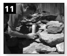
Black foam fills voids in the rockwork and forces water to run over the rocks instead of beneath and between them.
