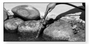
Fill the pond with water and check for leaks. Initially the pond may be cloudy from the accumulated debris of rockwork and dust. Over the course of a few days this debris will settle and the pond will gradually clear.
