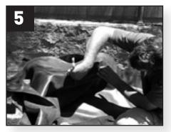
Mark position of the weir opening by rubbing the liner with a hard object such as a screwdriver or a blunt scissor edge.
