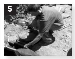
Place the Skimmerfilter<sup>™</sup> in the hole. Verify that the face of the Skimmerfilter<sup>™</sup> is flush with the back wall of the lined coping shelf.
