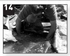
Position pond liner over the Skimmerfilter™ mouth and hold it in place. Smooth liner free of wrinkles and folds. Wipe clean.
