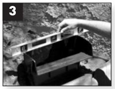
Place the Waterfall Weir<sup>™</sup> and level the unit front to back and side to side.
