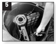
Lower pump into skimmerfilter chamber
