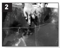
With pond full, mark position of water level on the liner at the Skimmerfilter<sup>TM</sup> location with white chalk.
