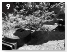
Backfill around the Skimmerfilter™ with the lid in place. Use moist sand or pea gravel, if this is unavailable, use gravel and loose soil (free from clumps).
