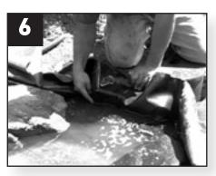
Check to make sure the water level meets the skimmer 3%" inches below the top of the neck. Adjust up or down by adding or removing soil.
