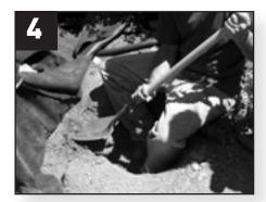
Dig a channel 7" below the water line, measuring 15" wide, from the hole to the pond. The Skimmerfilter™ neck rests on this channel. Compact and level the bottom of excavation. Do not dig too deeply or the soil may settle unevenly.
