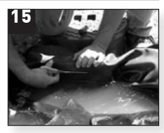
Make a 3" wide incision through the centered liner 3/4" below the top of the Skimmerfilter™ opening.
