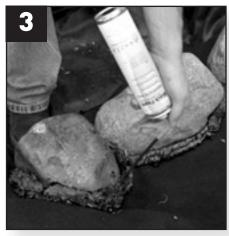
Use a bead of black foam to secure and seal the base of the rockwork.
