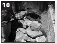
The final result with rockwork in place. Note: the rock running up the sides of the waterfall will be backfilled to hide the liner later on.
