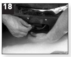
After the faceplate is properly tightened use a knife to trim the liner inside the mouth of the Skimmerfilter.™
