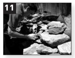
Black foam fills voids in the rockwork and forces water to run over the rocks instead of beneath and between them.
