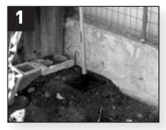
Level the soil in the area where the assembly is to be placed. Use blocks to add height to the waterfall.
