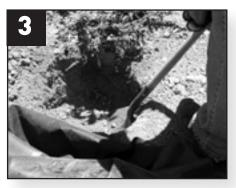
Dig a hole for the Skimmerfilter<sup> $\mathbb{T}$ </sup> in the previously determined spot. Place the hole 4" back from the coping shelf, measuring 24" across, with a depth of 14" below the marked water line.
