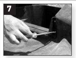
Attach liner bracket and liner to waterfall weir by installing 4 tack screws **halfway** into each corner. (Front of seal has recessed screw holes.)
