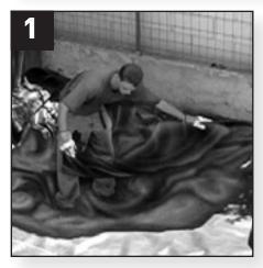
Place scrap underlay to protect the liner from abrasion and sharp edges.
