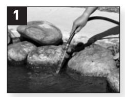
Fill the pond with water to accurately determine water level on all sides before installing the Skimmerfilter.™ Water level should hit partway up the coping stones. Verify that the water level is a few inches below the edge of the liner on all sides.
