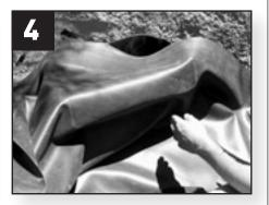
Place liner over the face of the waterfall. Leave a moderate amount of slack in the material.
