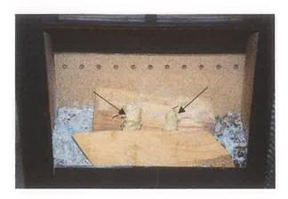
2. Start to build a lattice of stocks above the firelighters so that the flames from the fire lighters can easily pass through the sticks. This allows the most rapid heating up of the flue and produces less polluting flue gases during the warming up period.
