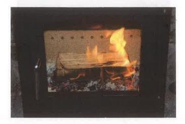
8. A correctly burning Si wood stove will "gassify" the wood. The intense heat within the combustion chamber and from the glowing charcoal base will drive out the gases from within the wood and create a very hot, clean burn which will deliver maximum heat from the wood whilst minimising the rate at which the wood is consumed. This is achieved on lower and medium burn rates and will produce a flame picture like the one shown below.
