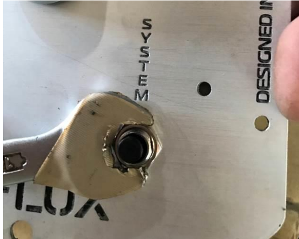
Figure 14: Replacing Overload Protector
