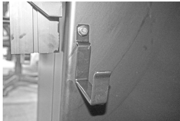
Fence Hook Installation
