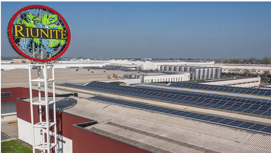
The Riunite production facility in Campegine, Reggio Emilia. Riunite is by far the biggest producer in Italy, with the closest competitor some 100 million bottles behind.
