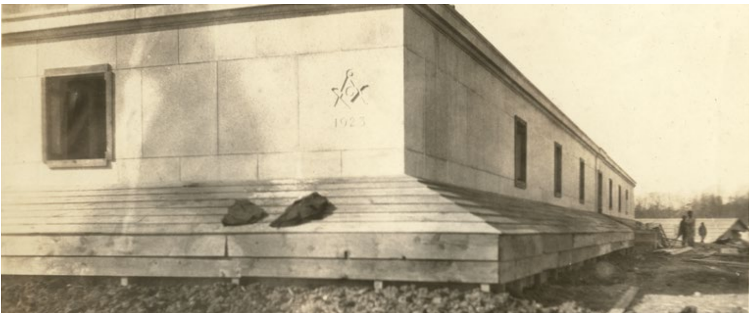
November 20, 1923. Less than a month after the cornerstone's ceremony, it was secure within the Memorial's east and north walls. Protective sloped wood covers were employed to prevent rainfall from flowing into the foundation.
