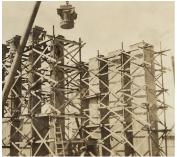
On April 7, 1925, the last of the capitals of Memorial Hall’s eight marble columns is installed. Wooden crates were built around each pillar and capital for protection as the Memorial was built around them.
