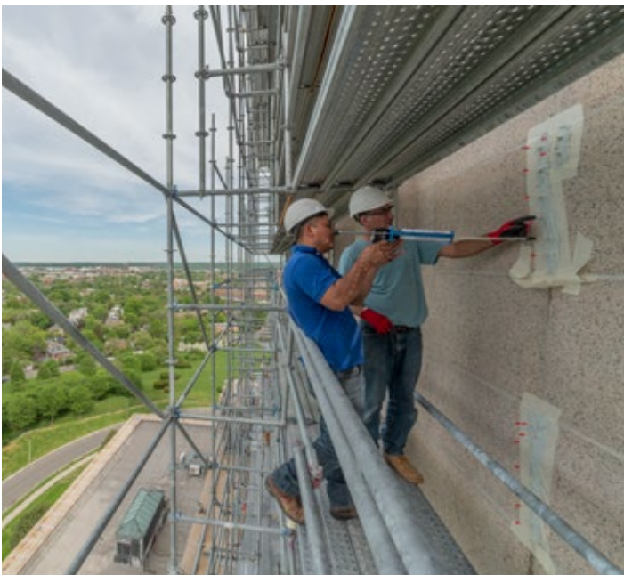
Stonemasons on the Memorial's fourth floor repairing cracks in the granite.
