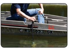
8. To install diffuser, loop a rope around 9. Once in place on the pond bottom, let go of one end of the rope and pull the other end until free to retrieve the rope.
