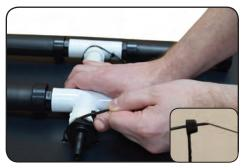
4. Secure assembly to underlay plate with supplied zip ties. Be sure to run the end of the zip tie through the correct side as shown.
